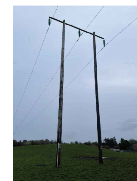
PYLON NO. 10 ESTIMATED HEIGHT: 12.4m
