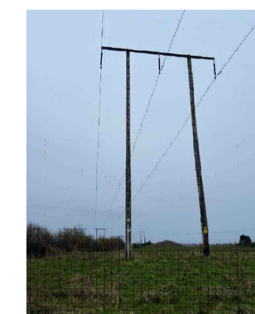
PYLON NO. 11 ESTIMATED HEIGHT: 11m
