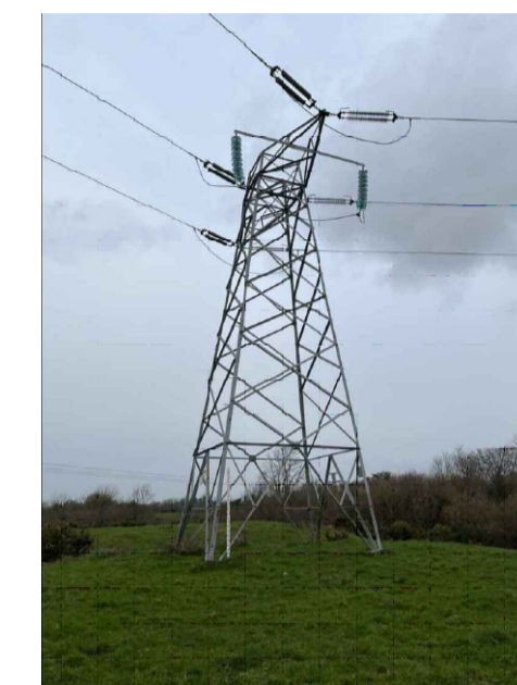
PYLON NO. 4 ESTIMATED HEIGHT: 10m
