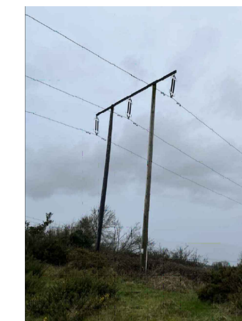
PYLON NO. 5 ESTIMATED HEIGHT: 12.3m
