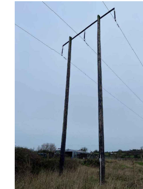
PYLON NO. 2 ESTIMATED HEIGHT: 11m
