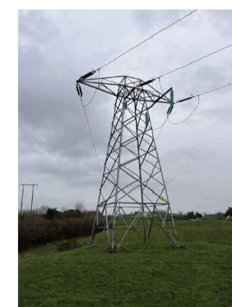
PYLON NO. 9 ESTIMATED HEIGHT: 10m
